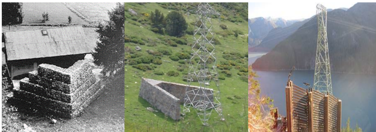
Figure 9. Avalanche Splitters made with different construction materials to deflect the course of the flowing avalanche [ANENA, 1994].
