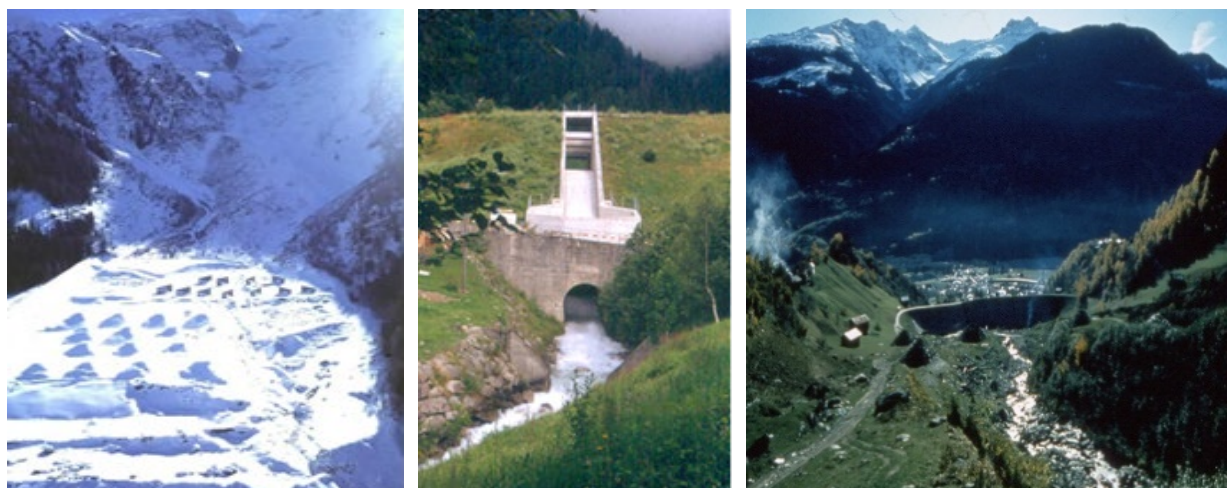
Figure 8. Avalanche protective dams in France and Switzerland to dissipate the flowing avalanche, to stop the avalanche and use summer water [SFISAR, 1992; ANENA, 1994].
