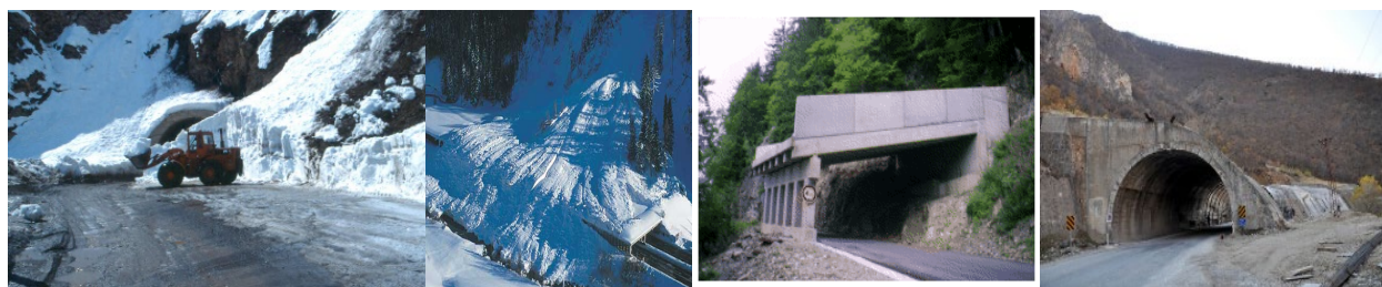
Figure 11. Avalanche tunnel at Van-Hakkar Highway [Gürer, 1993] and operational problems met (some of the tunnels on the Tunceli-Erzincan highway are being extended longitudinally) 2 .
