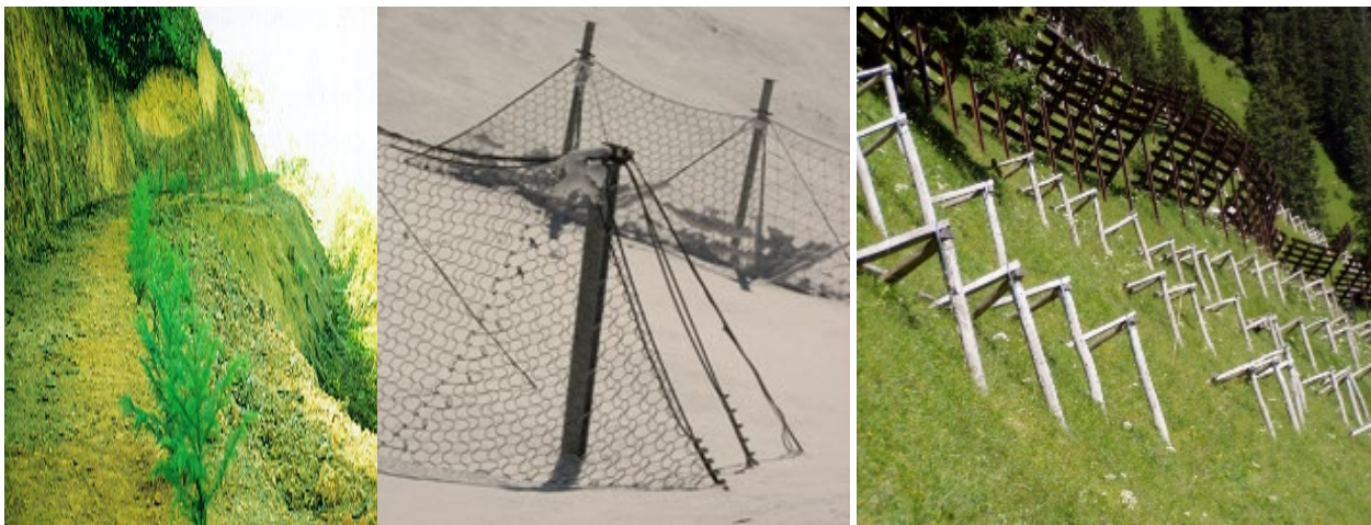
Figure 10. In the avalanche starting zone: Terracing, Tripods, Barriers, Avalanche Nets [Snow avalanches..., 1961; SFISAR, 1992; Gürer, 2015].
